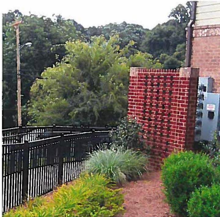
Figure 6-7-5 Service area screening
