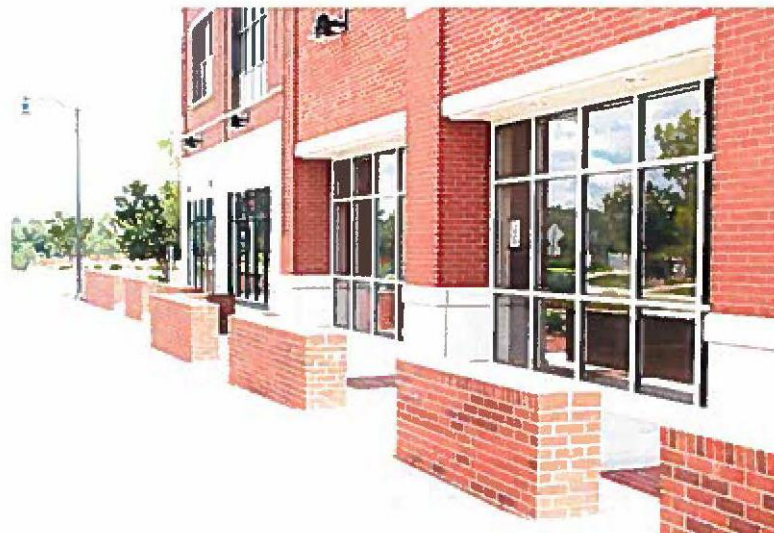
Figure 6-6-6: Facade transparency (windows) along a street facade
